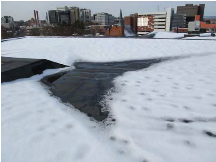
Adhered rubber membrane roofing on flat roof sections also replaced in recent years
