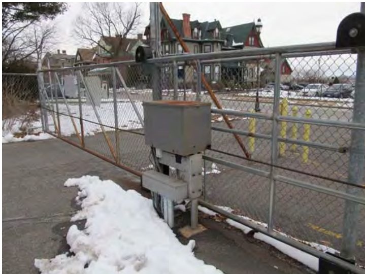
Motorized gate controls access to parking area
