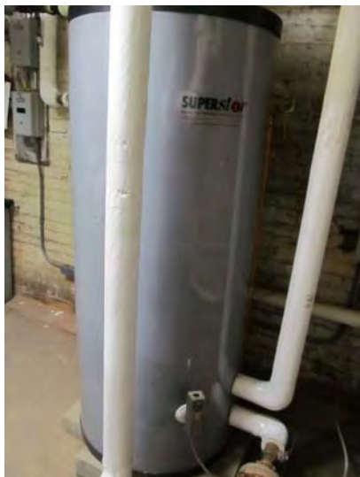
Freestanding, indirect-fired, domestic hot water tank provides storage capacity for the system
