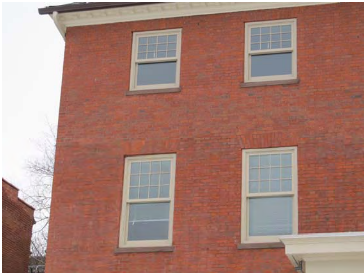
Exterior brickwork was recently re-pointed, and new windows were recently installed throughout the building
