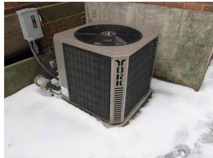
Exterior condenser unit for cooling of select areas at the first floor level of the building
