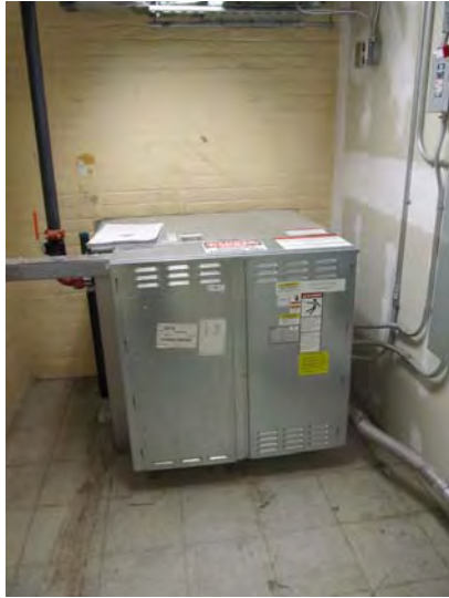
Hydro-mechanical and controller/dispatcher equipment for recently installed elevator that serves all floor levels of the facility
