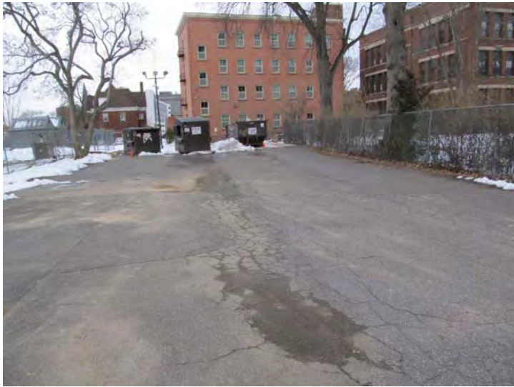
Asphalt paving at parking area exhibits age-related cracks and deterioration
