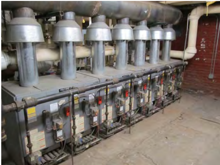
Hydrotherm natural gas-fired modular boiler plant for production of hydronic heat and domestic hot water
