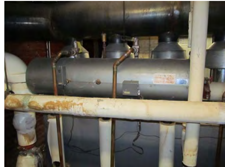
Hydrotherm shell and tube heat exchanger that works in concert with the boiler plant to produce domestic hot water for the facility
