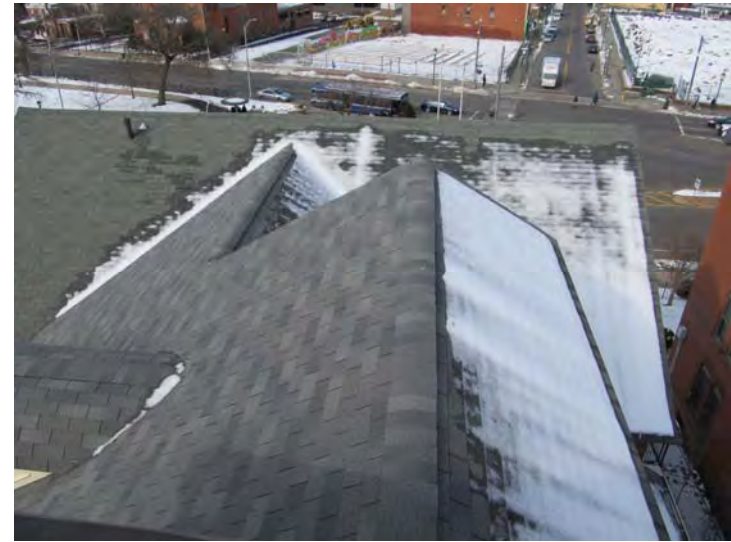
Shingles on pitched roof sections have been replaced in recent years
